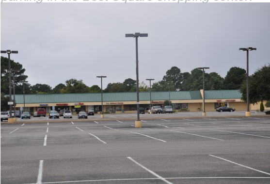
This image illustrates the over abundance of parking in the Best Square shopping center.
