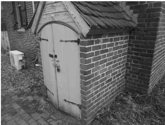
The shed to the ADU was locked with no access
