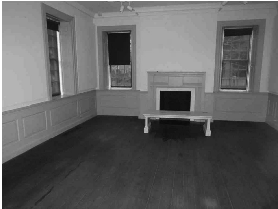
Living Room. Average flooring, and it appears mostly original.
