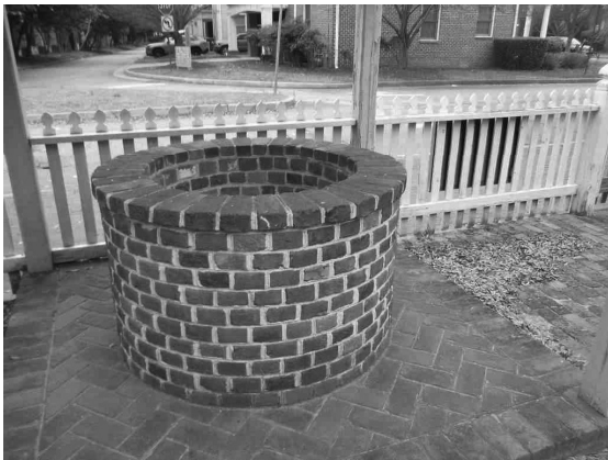
The well is non-functional
