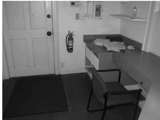
Office area. This area could be the kitchen (there is currently no kitchen in the main residence)
