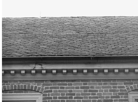
Custom millwork on the exterior, but the paint is in Fair condition. Roof appears to be a cement shingle
