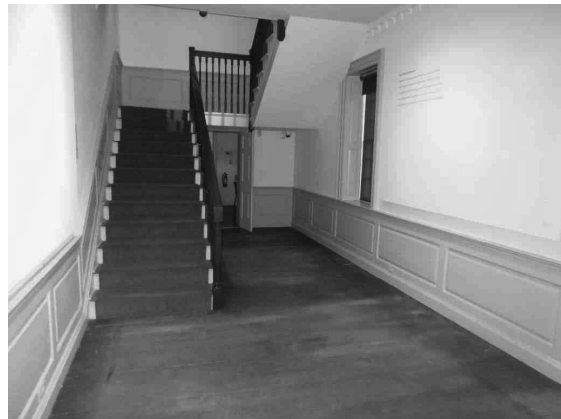
Entrance. Flooring and millwork appear mostly original
