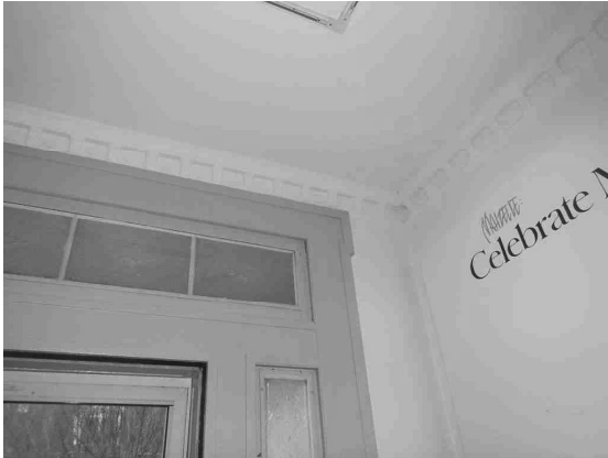
More custom millwork
