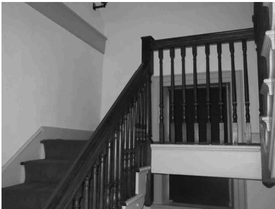
Stairwell to the third floor / attic
